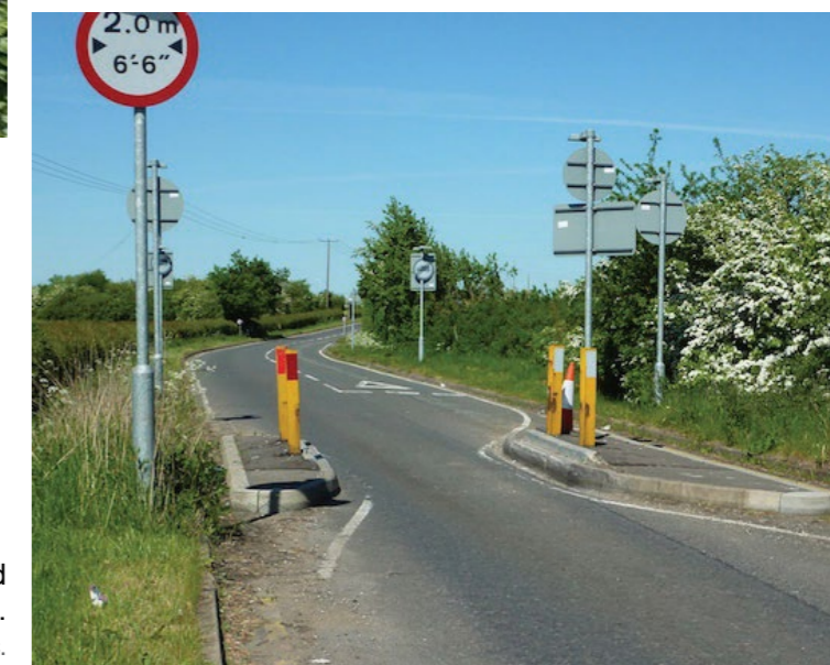
Right: Local Road Narrowing and Traffic calming solutions. Build outs are used here to slow down traffic.
